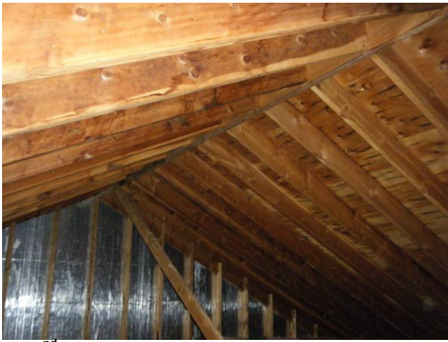
48 2 nd story attic space
