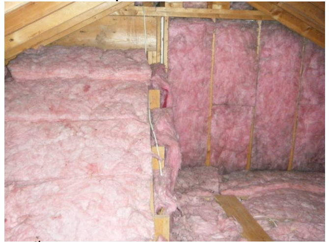
40 1 st floor attic space
