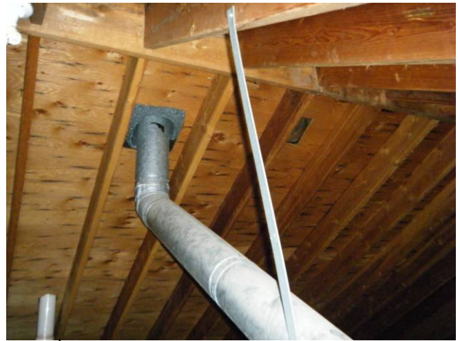
47 2 nd story attic space
