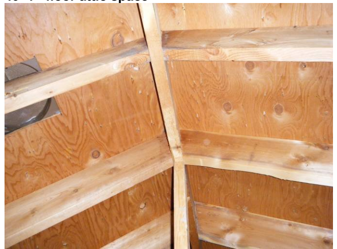
41 1 st floor attic space
