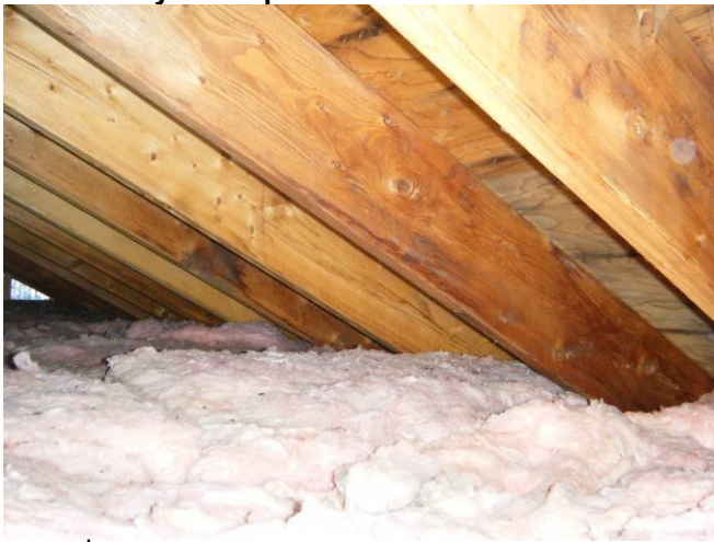
44 2 nd story attic space
