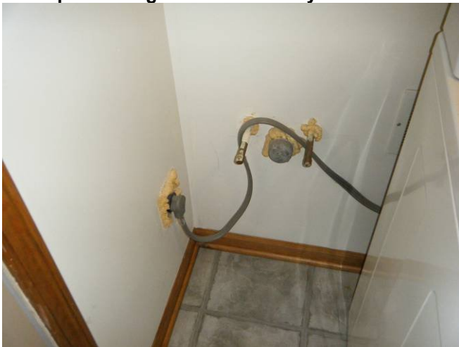
21 Utility sink hook-up
