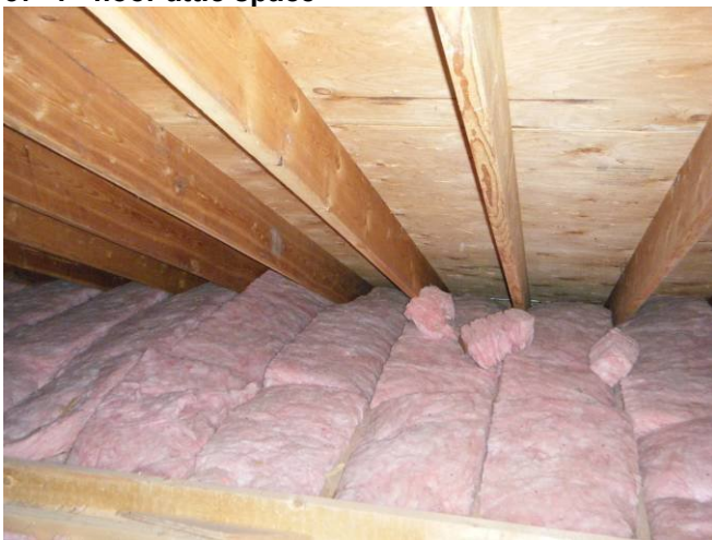
38 1 st floor attic space
