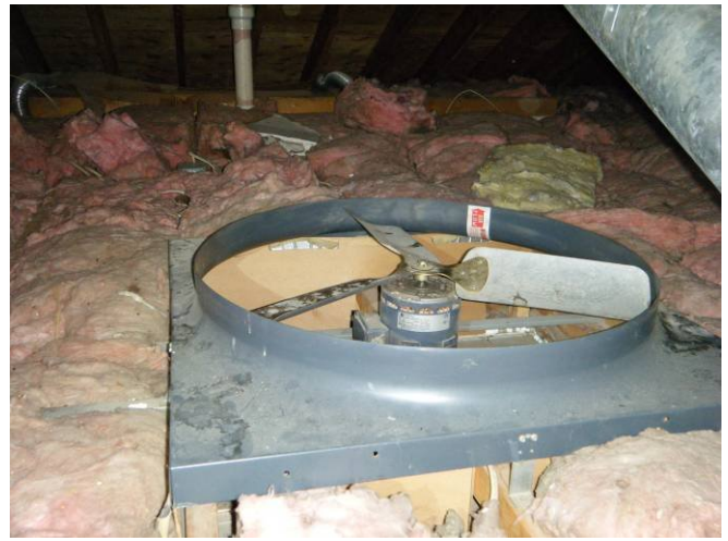
45 Seal and insulate fan in cold months
