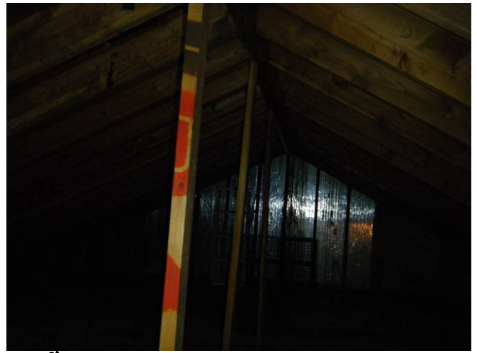
39 1 st floor attic space
