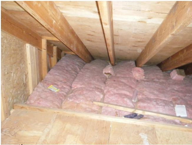
37 1 st floor attic space
